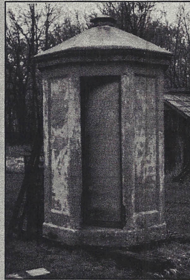
Victorian public park privy, (panelled door has been covered.).
