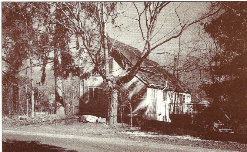
124 Georgetown Road. Gertrude Johnson moved to this house (now extensively renovated) at age 1. The house was built by her great uncle Adam Kennel.
