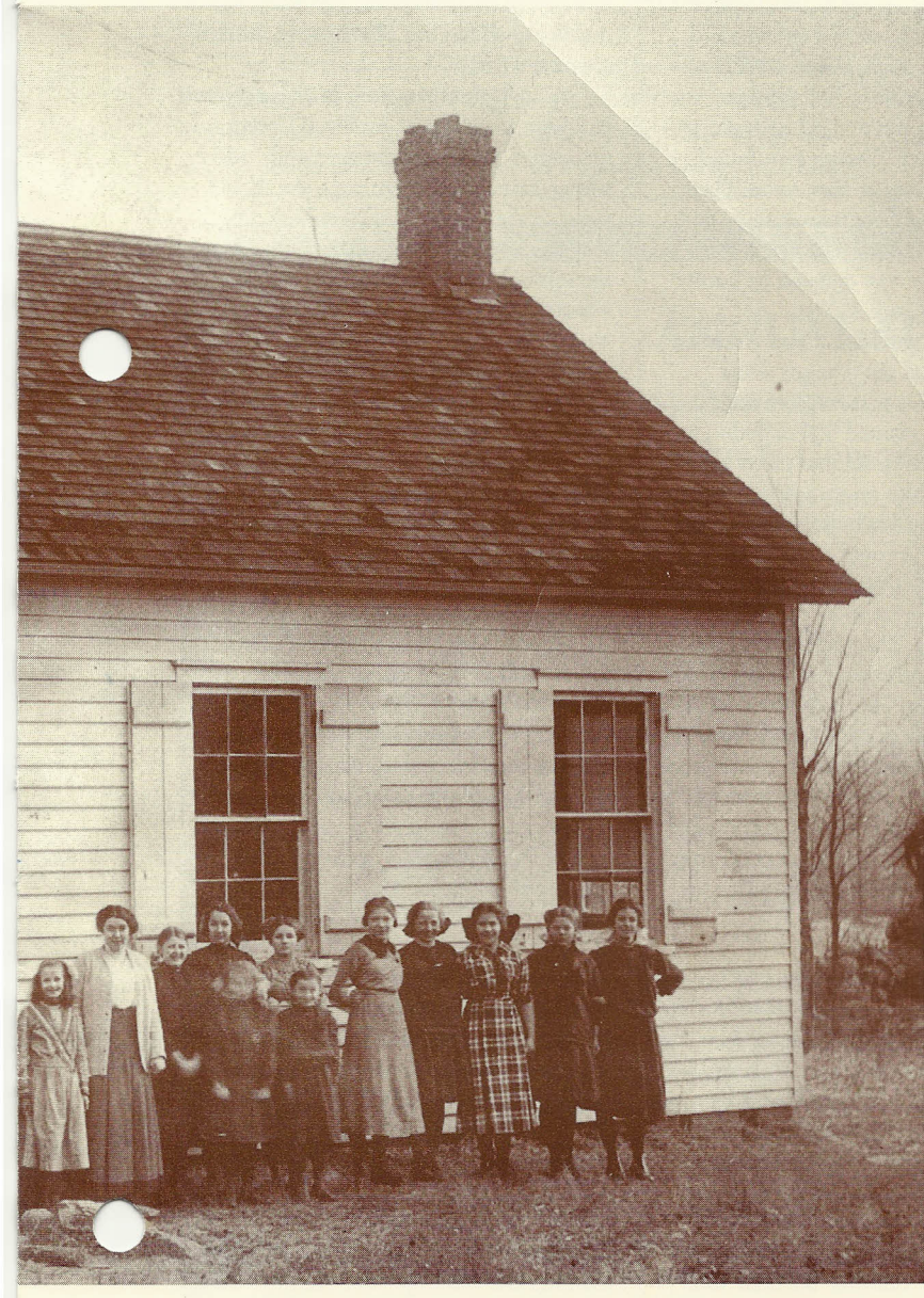
1928), located at 47 Godfrey Road West.
