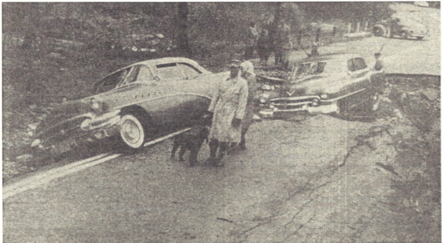
Weston Road Washout: Gullies cut by raging rainwater, into which the cars of Gerald Vosburgh and Arnold Bernhard stumbled in the driving rain Saturday night.
