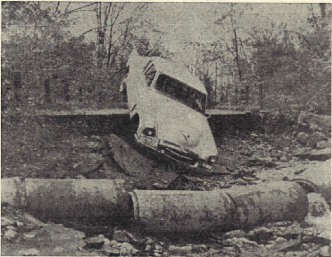
Norfield Road near Weston Road: An excellent example of the pitfalls into which motorists fell during the rain at the height of the storm.
